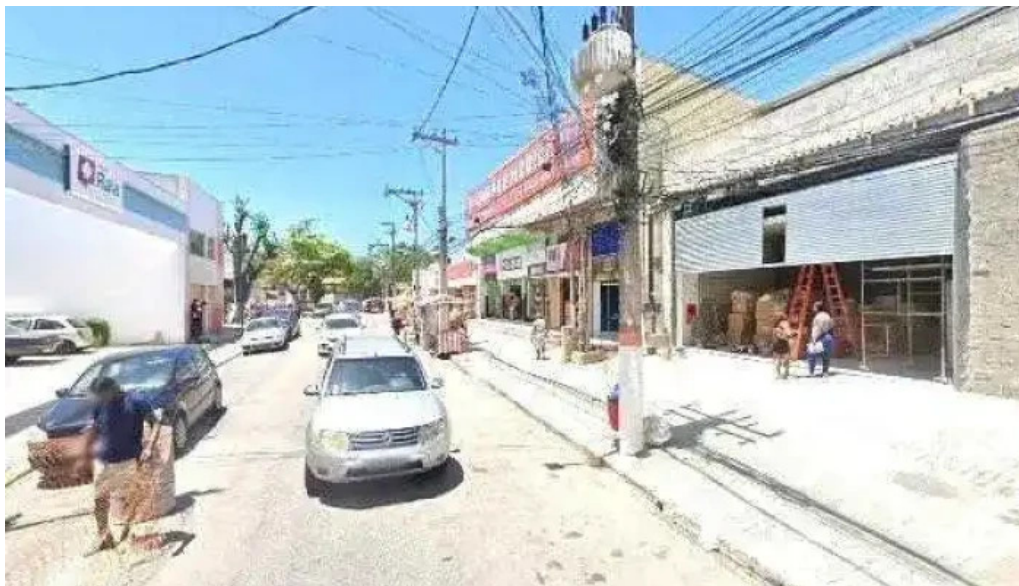
South co marica street view e 360deg
