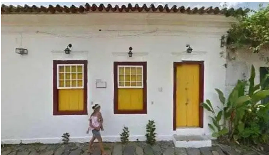
Celeiro armazem tropical street view e 360deg
